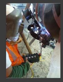
Orbital Gas Metal Arc Welding system to produce high quality welds.
