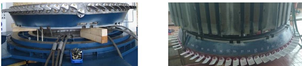
a) Upper row of ventilation ring vanes
