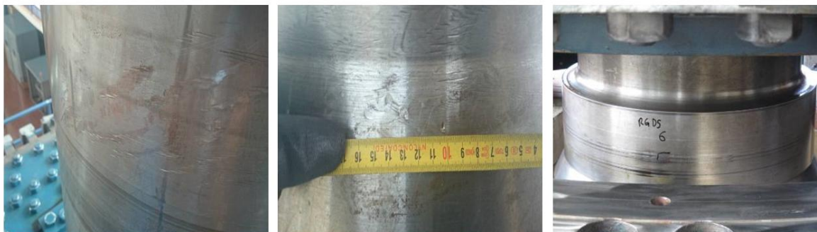
a) Appearance of mechanical damages in area 1
