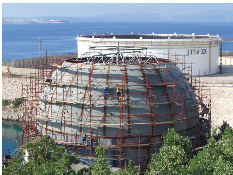
Figure 3. Segments of spherical tank positioned and welded together [3]
