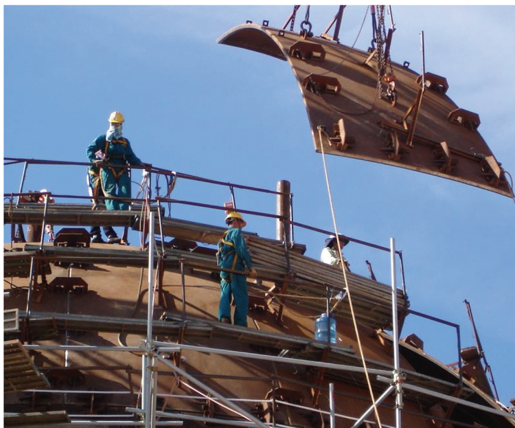
Figure 2. Segments of spherical tank are positioned and welded [2]
