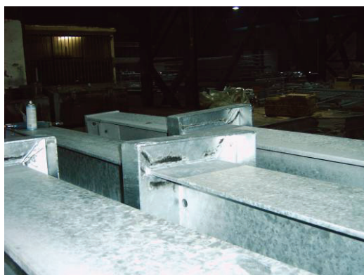
Figure 1. Example of zinc coating faults
