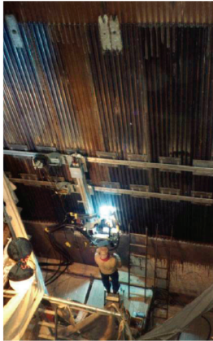
MAG welding of Ni-based alloys with CRONIGON® Ni10
