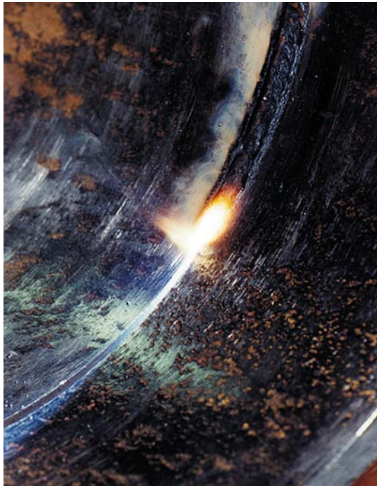
STT® root pass welding (Inside Pipe).
