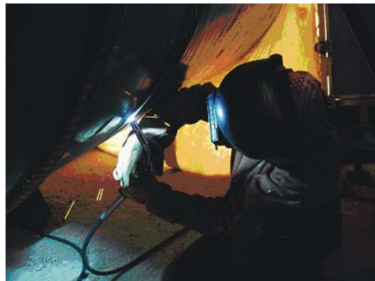
STT® root pass welding (Outside)
