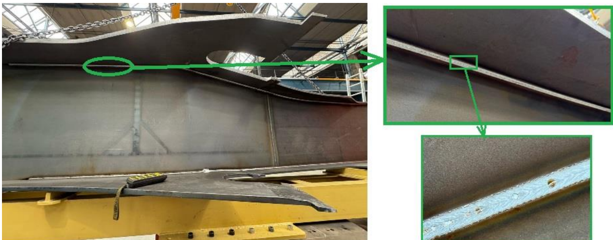
Figure 17. Weld a3 on the "S" beam
