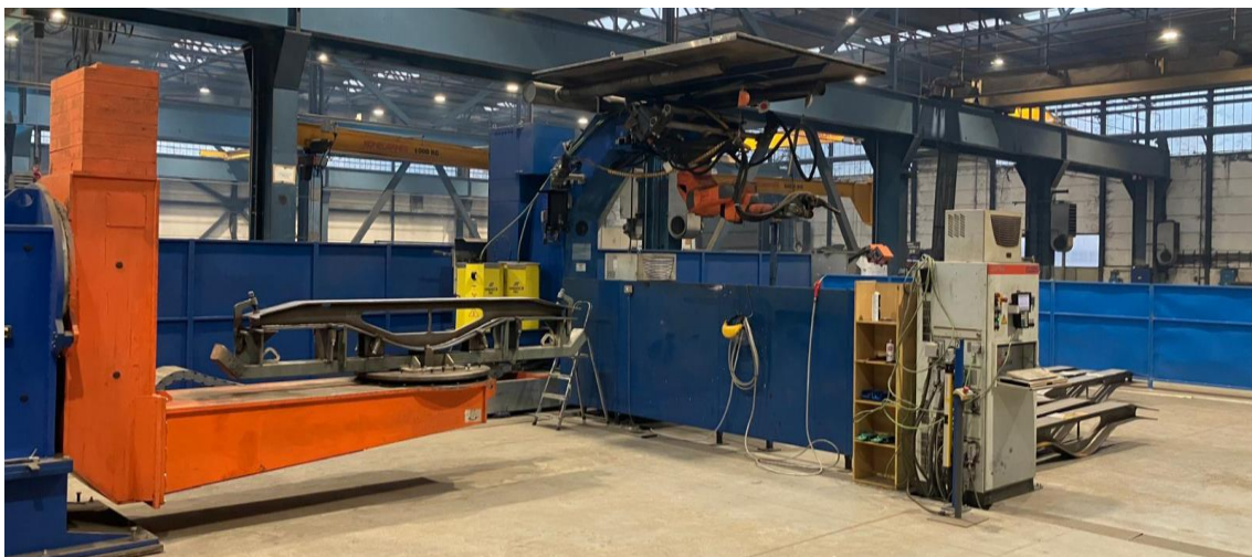
Figure 7. Robotic welding station Cloos QRC350
