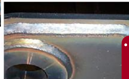
Example of good wire placement
